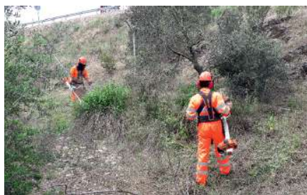
Figure 5: Clearing of hard shoulders.
